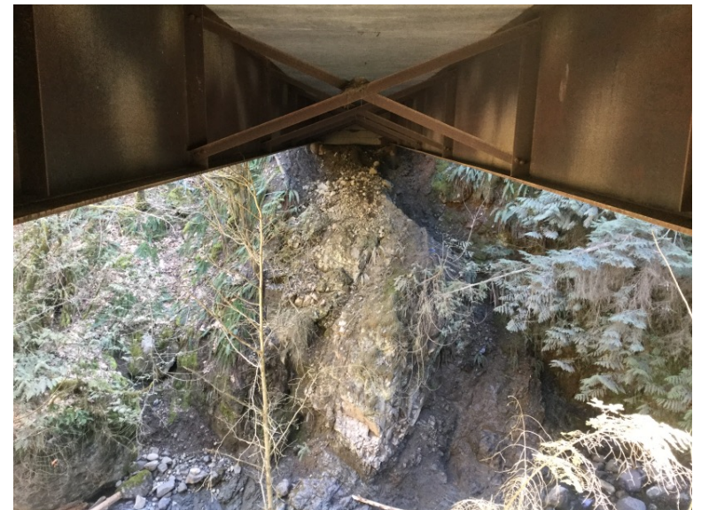
Right Bank Abutment when facing downstream
