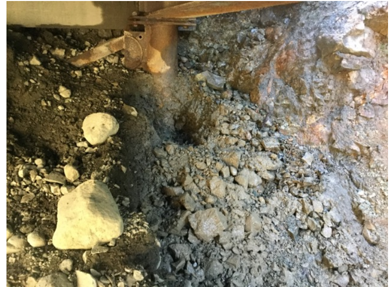
Upstream right bank fill condition
