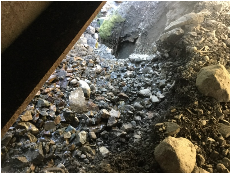
Upstream right bank fill condition
