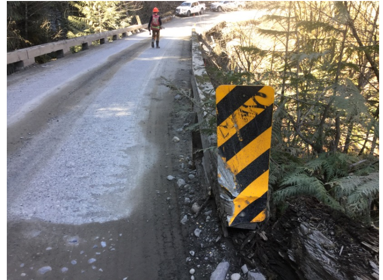
Downstream right bank guardrail condition
