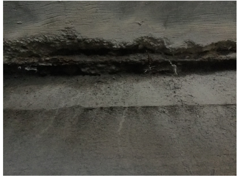
Underside of deck panel 1 at right bank
