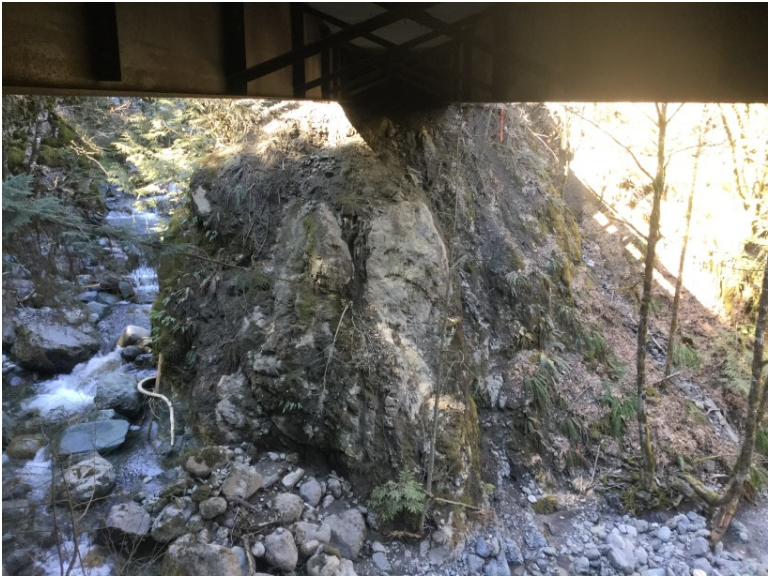
Left Bank Abutment when facing downstream
