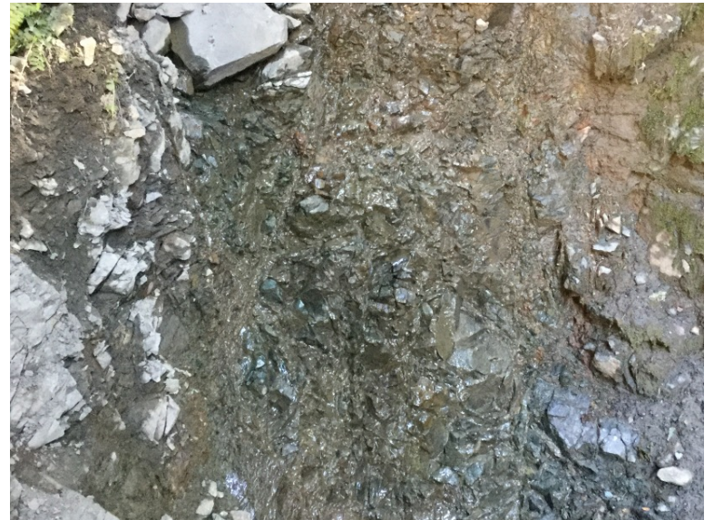
Parent material below upstream right bank pipe column
