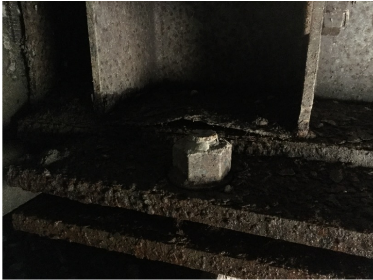
Right bank steel delamination
